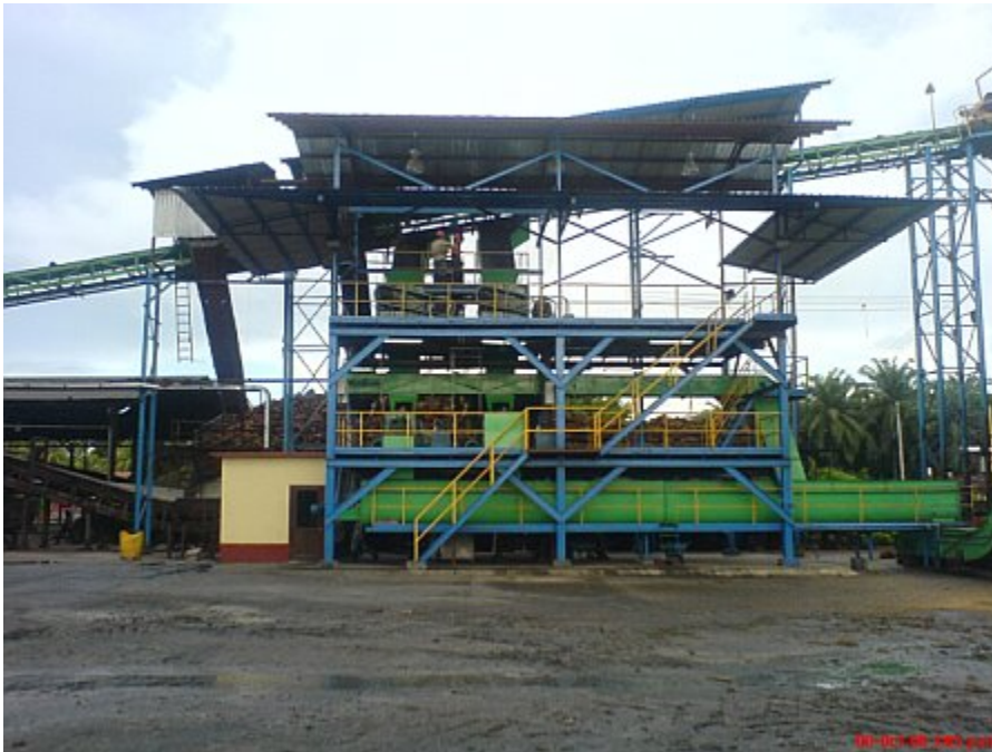
The Agrotor Biomass Plant
